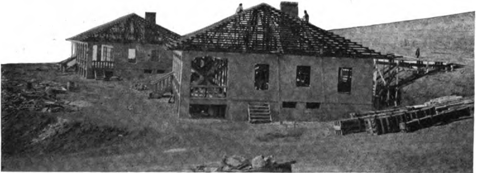
The Cottages for the Chief and Assistant Engineers at Marshalls are Nearing Completion
