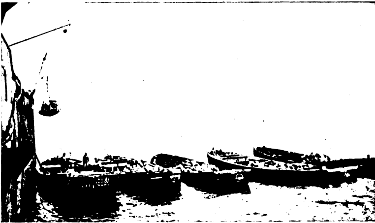
At Antofagasta the ship lay far out in the bay and the cargo was towed out in lighters and carried aboard by the ship's winches
