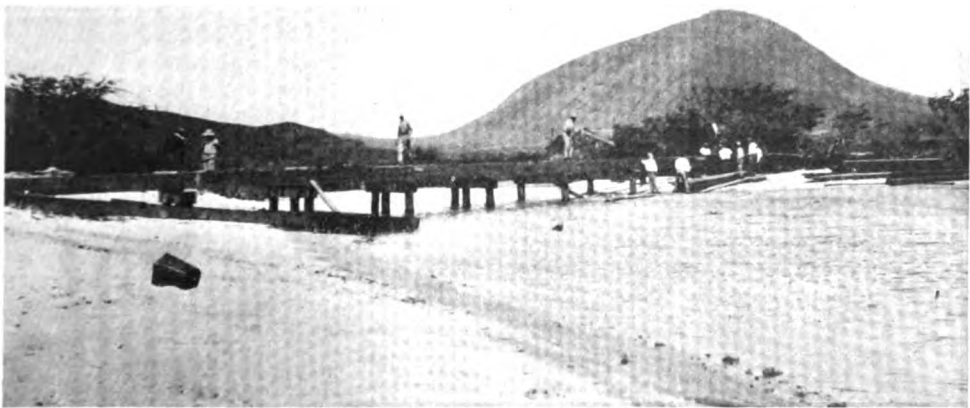
From disheartening experience transportation of materials to Koko Head by the sea route has proven neither safe nor speedy. Consequently the greater part of the material has been hauled to the site by road. When this was first tried in the midst of a tropical downpour the wagons slid sideways off the muddy roads and the material finally had to be brought piecemeal to its destination. The roads have been improved by regrading and the bridge shown in the photograph has been built across the pond.
