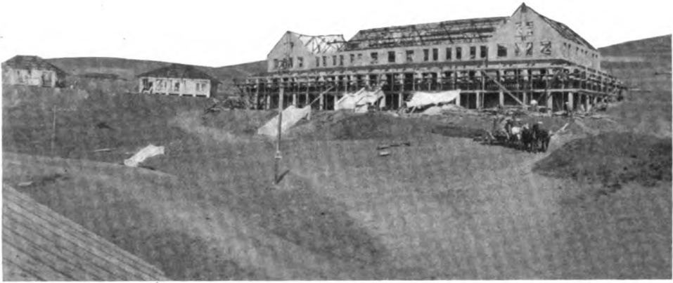
A panoramic view of the buildings in course of erection at Marshalls, Cal., where residences of the engineers; which the picture shows to be nearly complete, are located about from the
