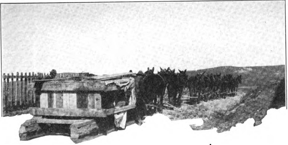
In attempting to negotiate this road on wheels a wagon had sunk almost out of sight and the machinery skids rested on the normal road level. The machinery was eventually rescued by one of the sledges built by the village smithy and pulled along the road by sixteen mules
