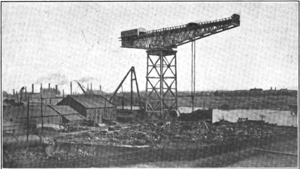
At Wallsend-on-Tyne the largest floating crane in the world lifted out our engine; every week a ship was launched somewhere within sight of us
