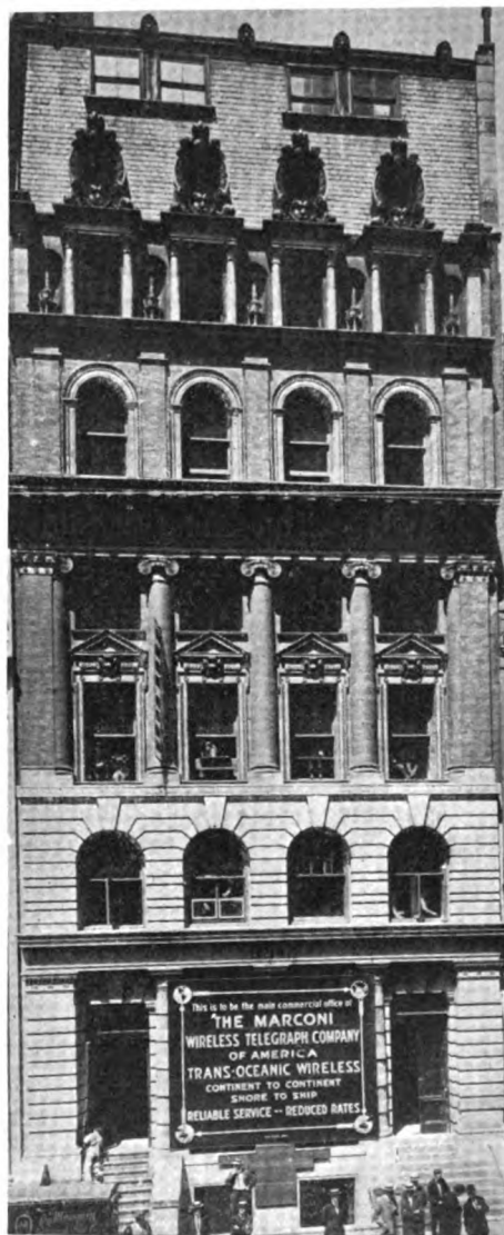
The Main Commercial Office is in the Heart of the Financial District, Occupying the First Floor of the Wall Street Journal Building on Broad Street
