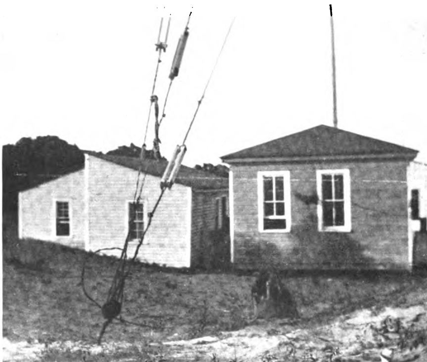
At the Marconi headquarters comfortable accommodations are provided for the operating staff in a separate house containing three bedrooms and a generously proportioned living room
