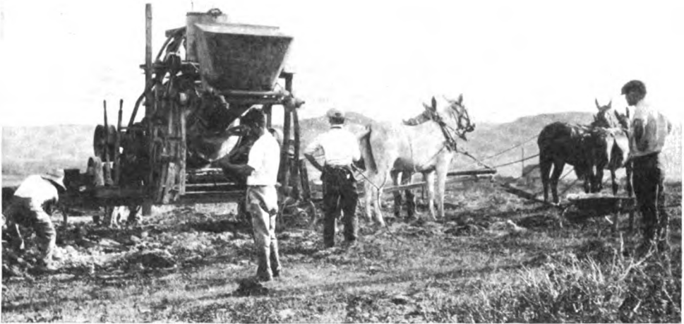
Motor trucks, which were used to haul material, made such slow progress, because of the condition of the roads during the rain, that horse-drawn vehicles were requisitioned to keep the field force supplied with material.
