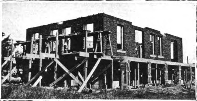
The Operating Building at New Brunswick, where all the Edifices combine sightliness with utility
