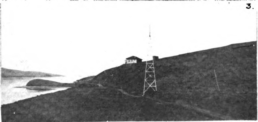
(1) A panoramic view of the California receiving station, showing the operators' hotel and the engineers' cottages. (2) A schooner driven ashore at the Bolinas site during a January gale. (3) One of the smaller towers for the aerial balancing lines.
